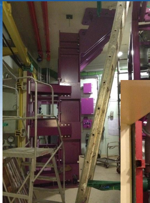
Underground door reinforcement
