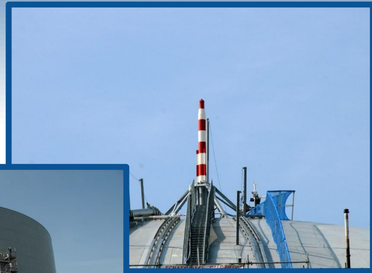
Emergency depressurization circuit chimney
