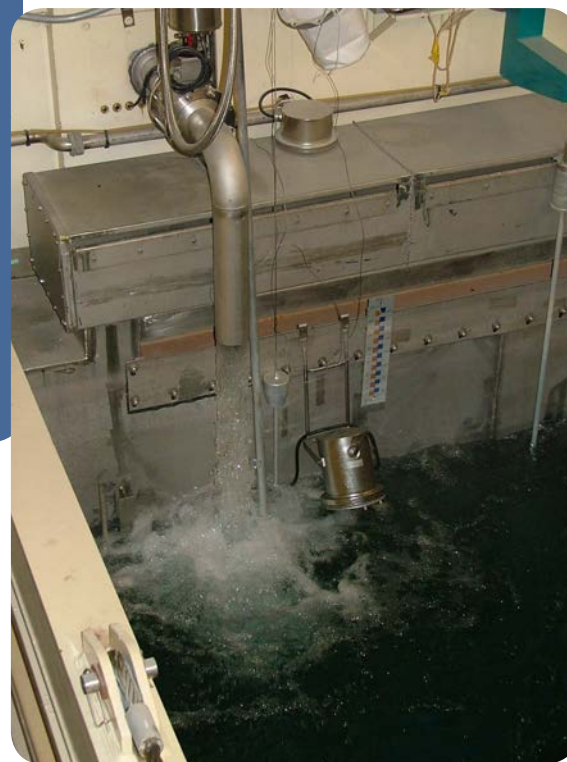
Emergency filling of the canal 2 containing spent fuel elements on level D (reactor pool level)
