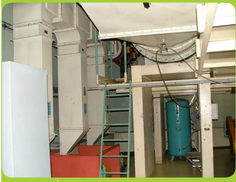
Air outlet of the reactor building ventilation system
