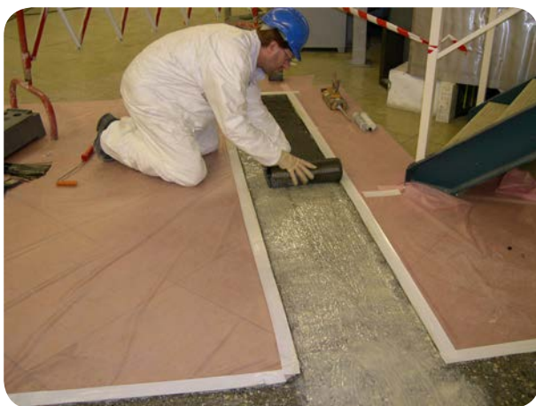
Laying and pasting of the fabric
