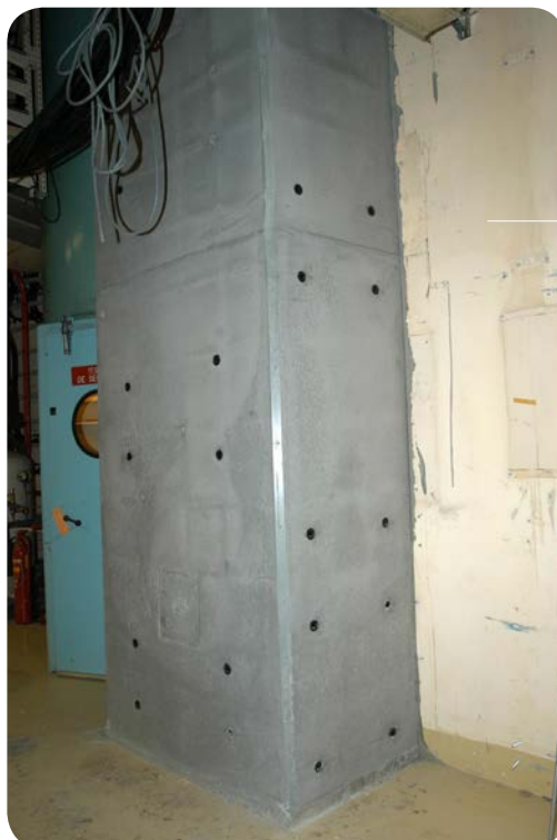
Reinforcement of concrete column under the back wall at level B (basement)
