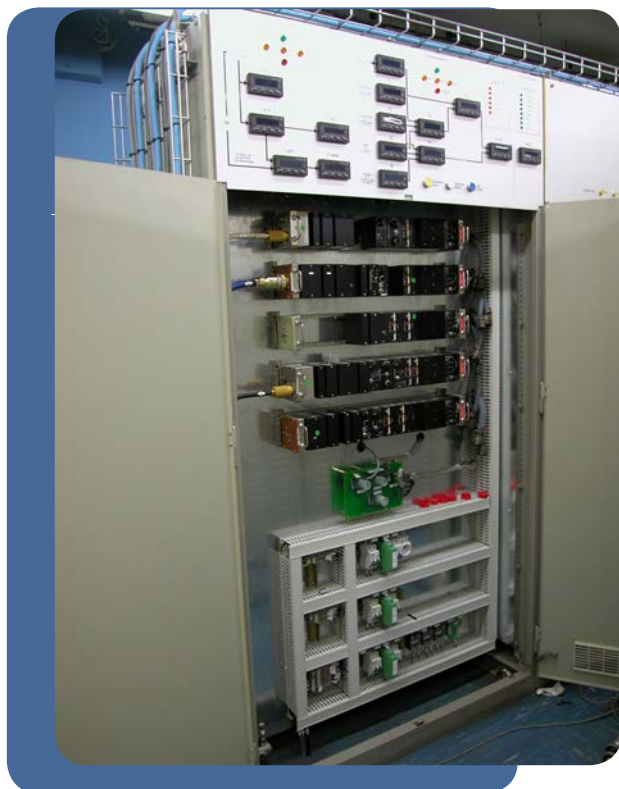
Reorganised cabinet for neutronic safety systems
