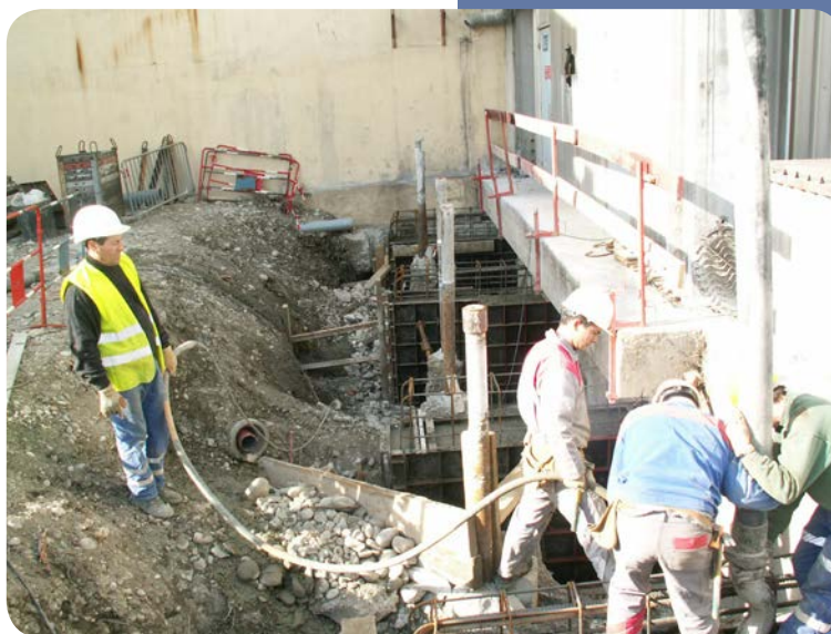
Adding micro foundation piles under the reactor air intake building
