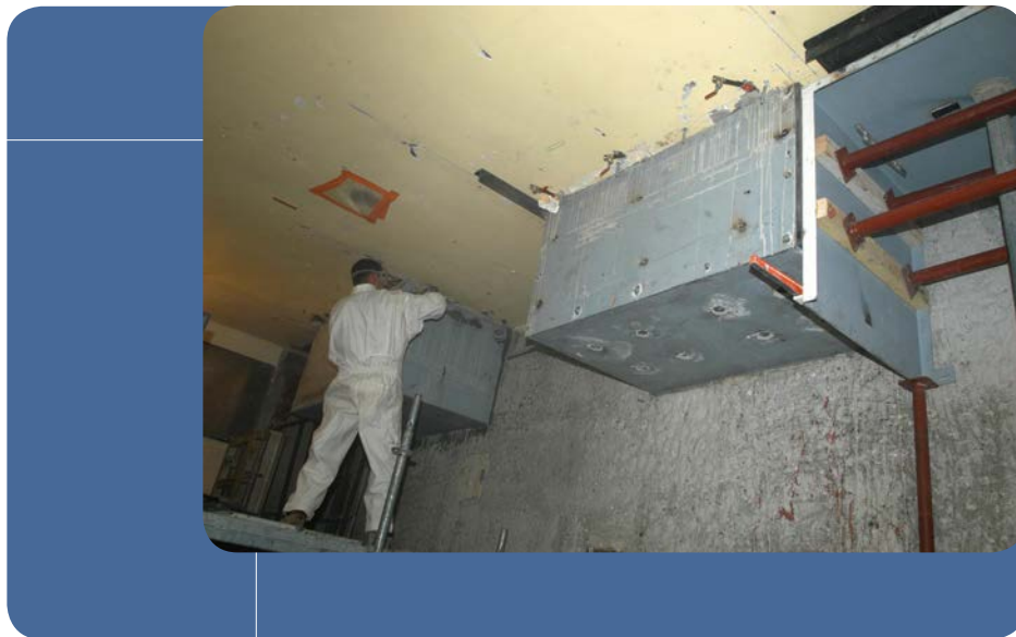
New cogs between level C (experimental hall) and level D (pool level)
