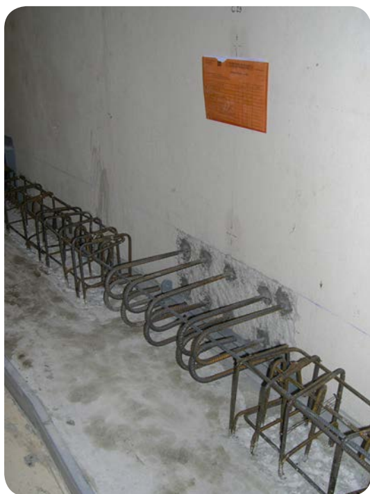
Steel framework for the 'comb'
