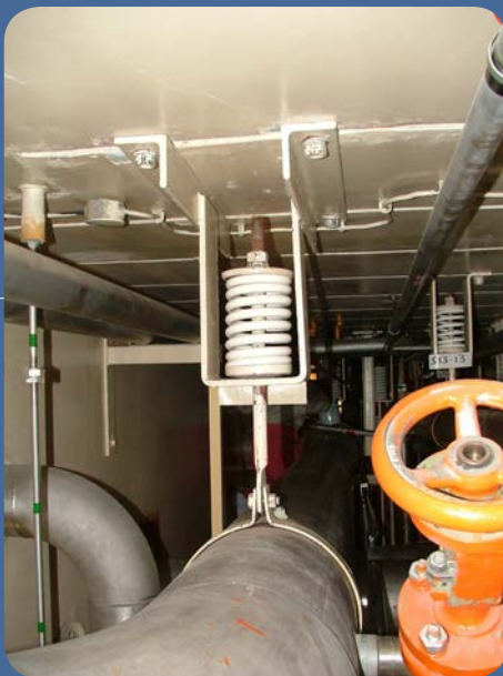
Renovation of pipe supports
