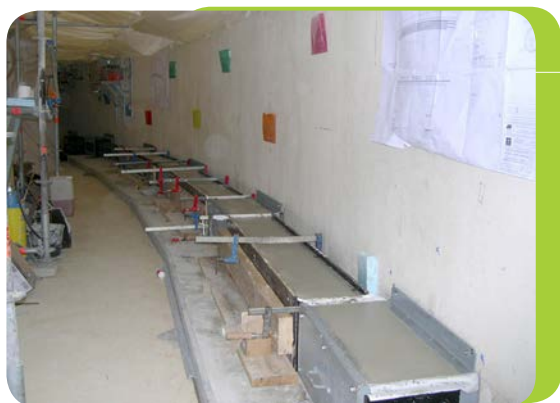
Concreting the steel framework
