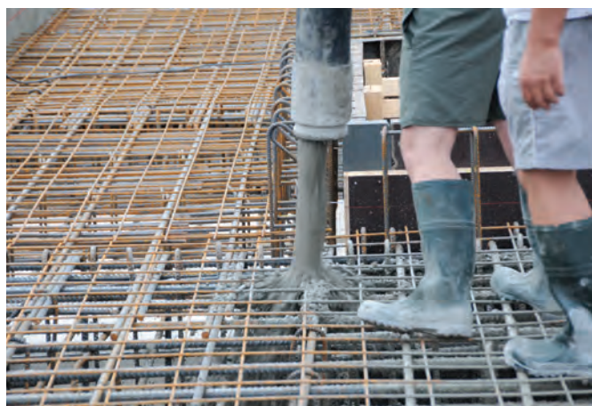
A forest of metal for foundations equivalent to those for a 50-storey building.
